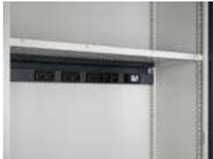
Raceway applied on the bottom part of the perforated shelf-panel
